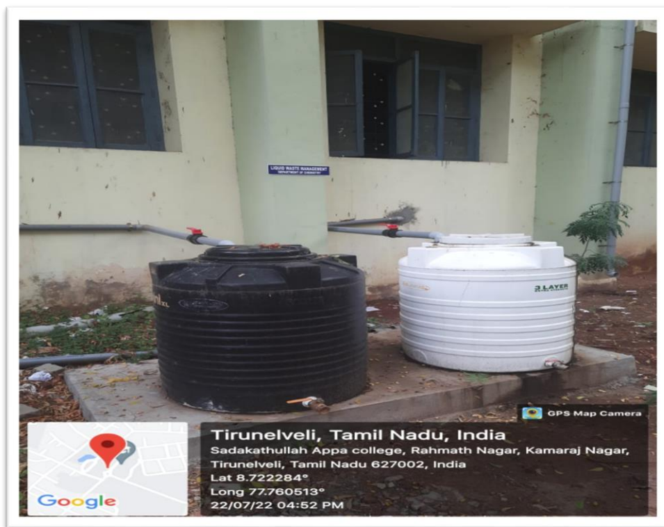
Liquid Waste Management Tank: Department of Chemistry
